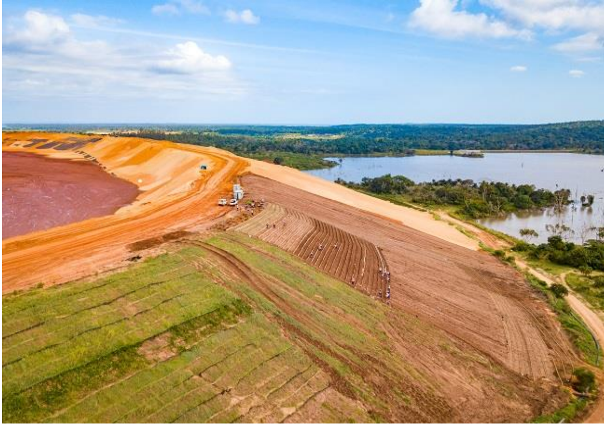
Base titanium tailings dam, 2017
